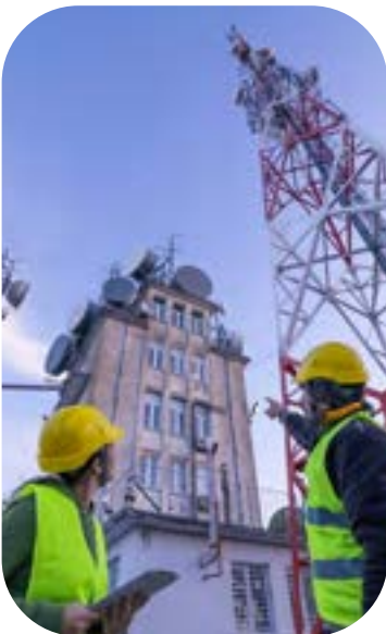
Wireless communications tower contracting
