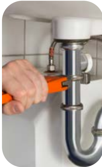
Plumbing and sanitary works
