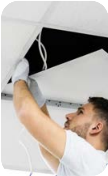
False Ceiling & Light Partitions works.
