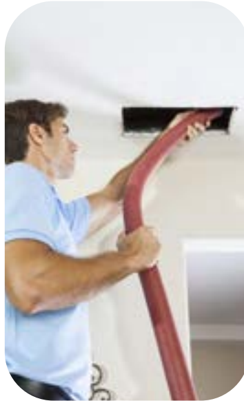
Air -condition duct cleaning Services
